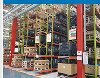
Very Narrow Aisle Pallet Racking System
