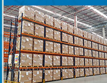
Selective Pallet Racking
